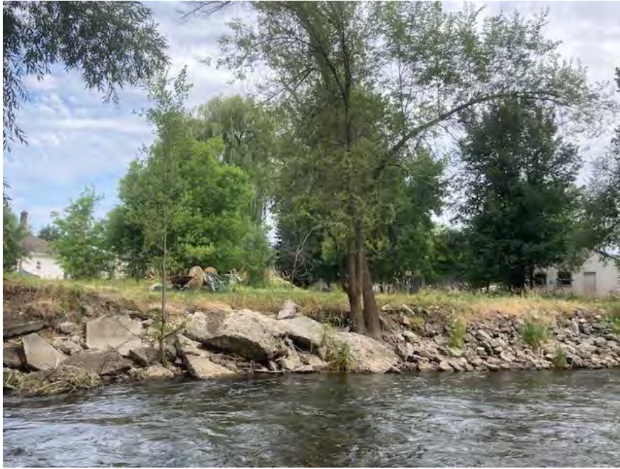
Photo 1 Degraded riverbank and riparian zone along the Logan River in API for Alternative 1 (north of the river alternative).
